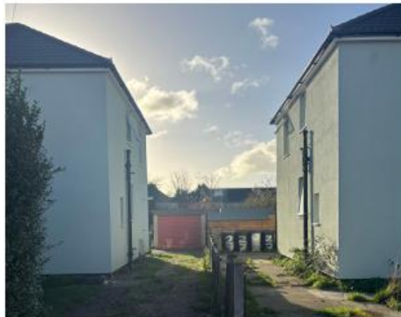
Fig 5. Nos. 23-27 King's Hedges Road, access between Nos. 25 i 27.
