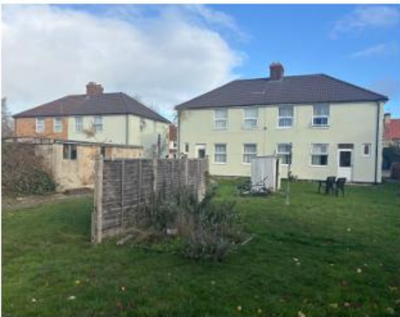
Fig 6. The Site Area - rear garden of Nos 23-27 King's Hedges Road, view of the rear elevations of the existing buildings.
